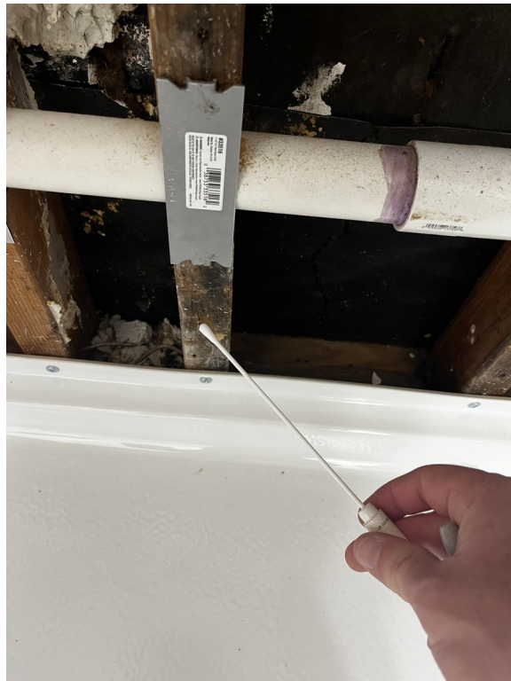
Photo 5: Unfinished bathroom — exposed wall framing, plumbing (PEX and PVC), and exterior sheathing behind the shower area during active remodel.
