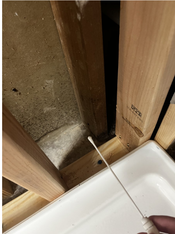
Photo 7: Close-up of lower wall cavity in unfinished bathroom — swab sampling area showing foundation and framing at tub base. Minor dust and debris observed; no visible active mold growth.
