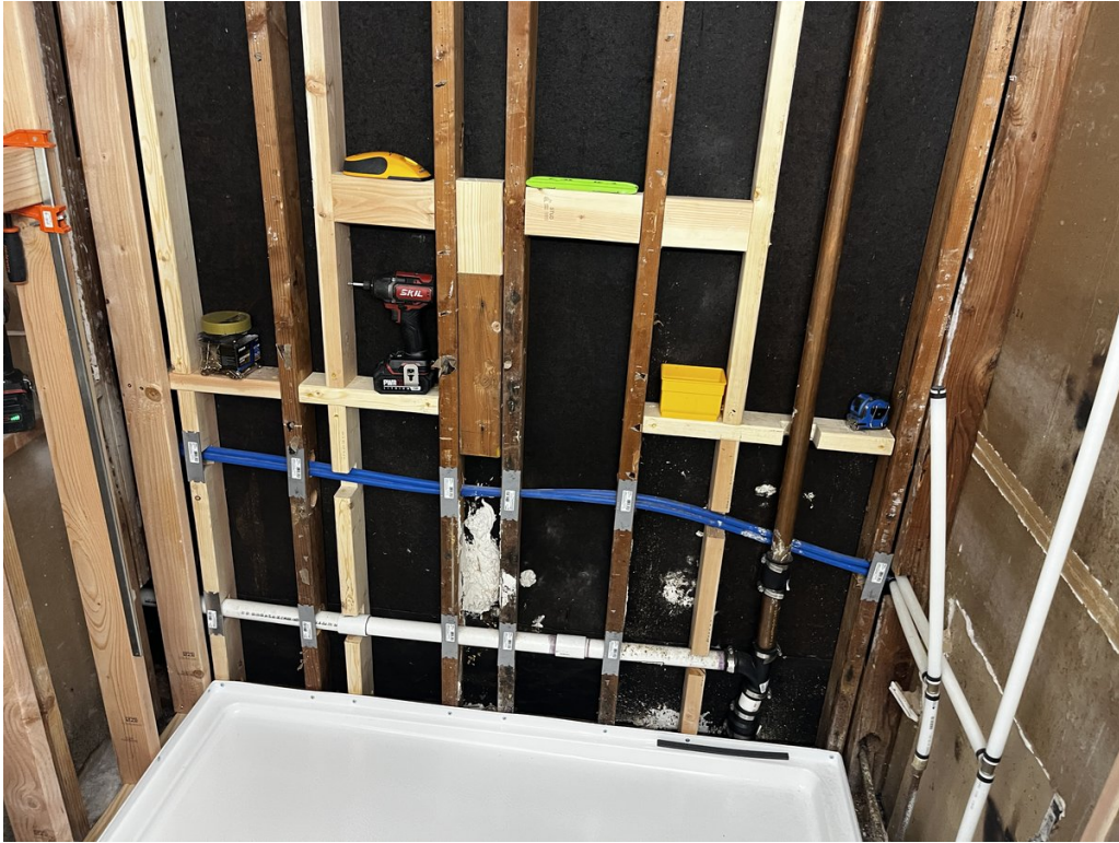
Photo 5: Unfinished bathroom — exposed wall framing, plumbing (PEX and PVC), and exterior sheathing behind the shower area during active remodel.
